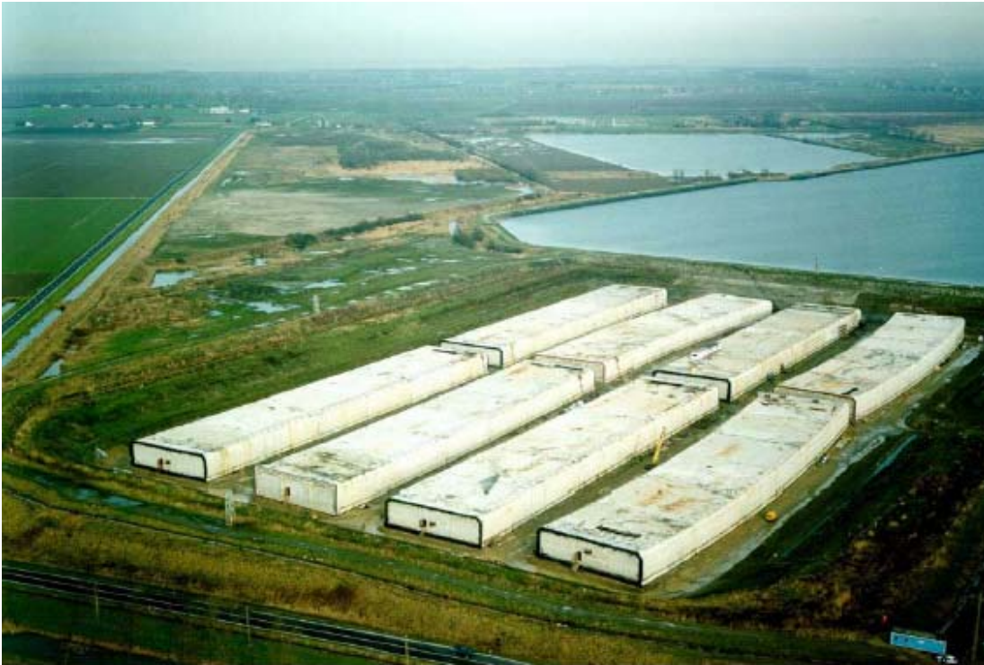
Elements prior to flooding of lagoon and launch
