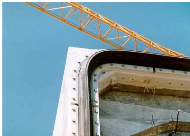
Submerged Tunnel Seal
