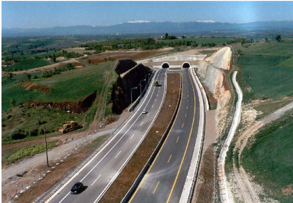
Tunnels constructed in hard rock, Greece
