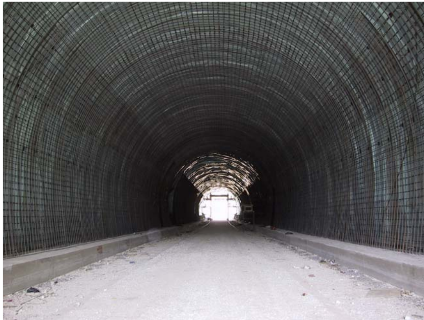
Reinforcement for Concrete Lining
